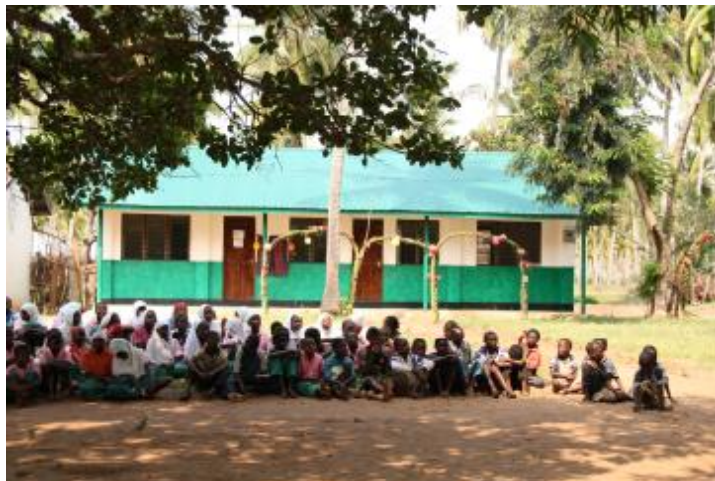
The new school building ready to open (Photo taken by a volunteer on Team 3)
